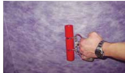
2. Embed Wall Seal with hand roller or straight edge.
