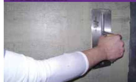
1. Apply bonding agent (NobleBond EXT or latex modified thin-set).
