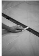
During the Re-Install Strainer Step - Position all strainers prior to fastening down with screws.
